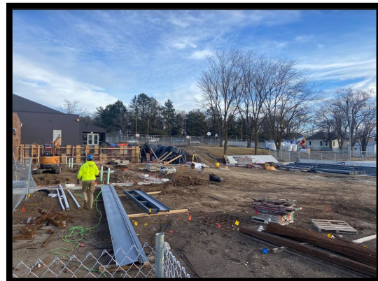
Bennet Elementary East addition facing North
